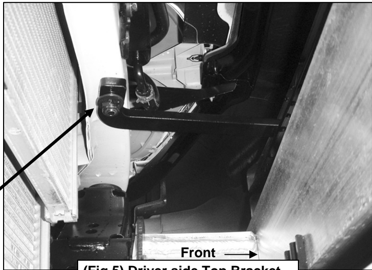
(Fig 5) Driver side Top Bracket installation pictured from below
